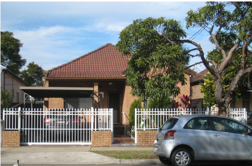
Photo 2: view of 20 Campsie Street, looking north from Campsie Street
