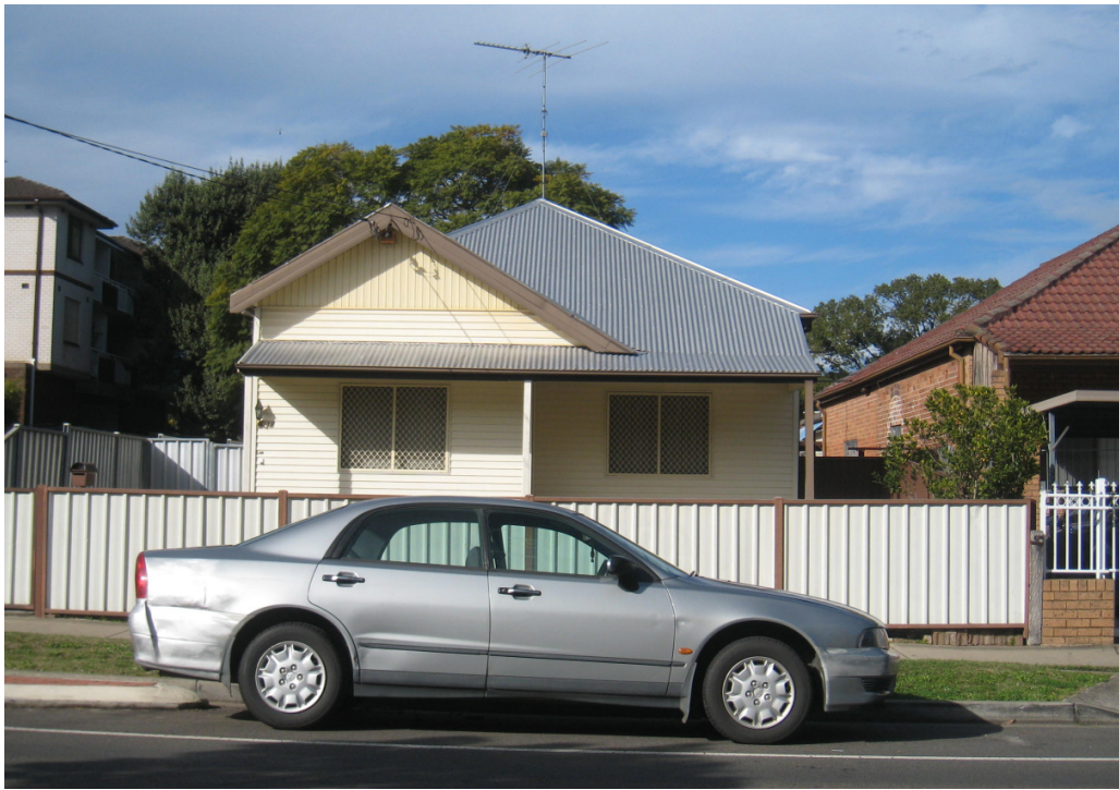
Photo 1: view of 18 Campsie Street, looking north from Campsie Street
